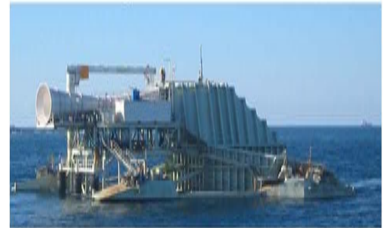
Oscillating Water Column Oceanlinx
