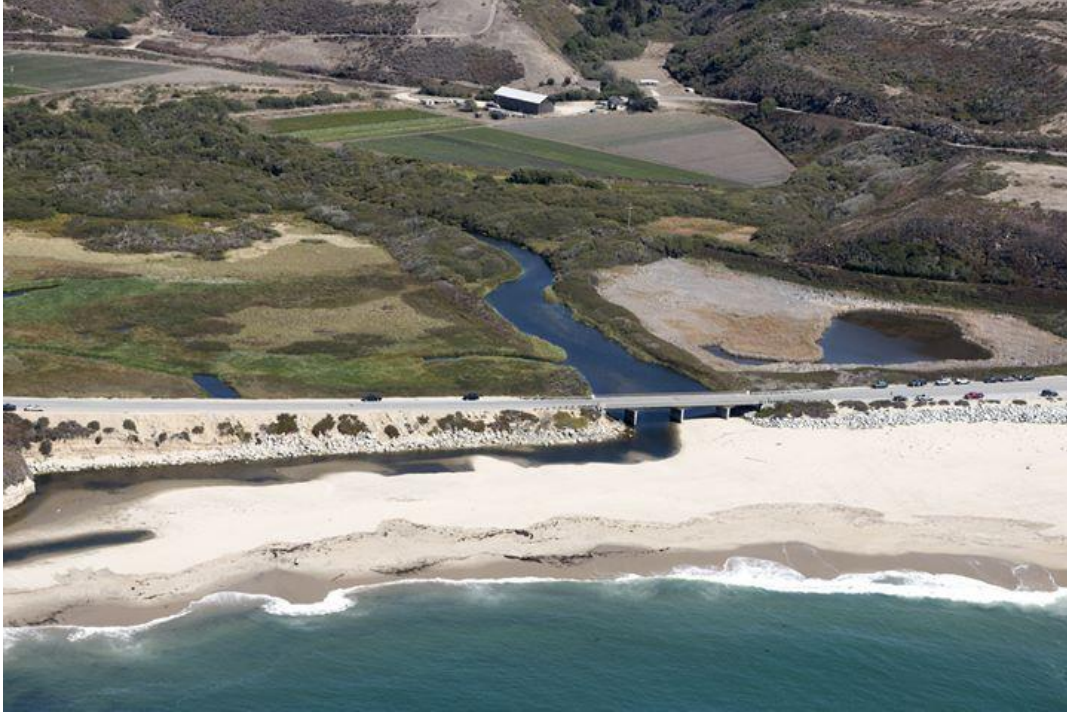
Figure 3-10. Aerial photograph of the Scott Creek Beach BECA and sediment impaired Scott Creek Lagoon, dated Sep 2010. The bridge and raised roadway constrict the mouth of Scott Creek and effectively isolate the lagoon from the open coast. Source: Adelman and Adelman.
