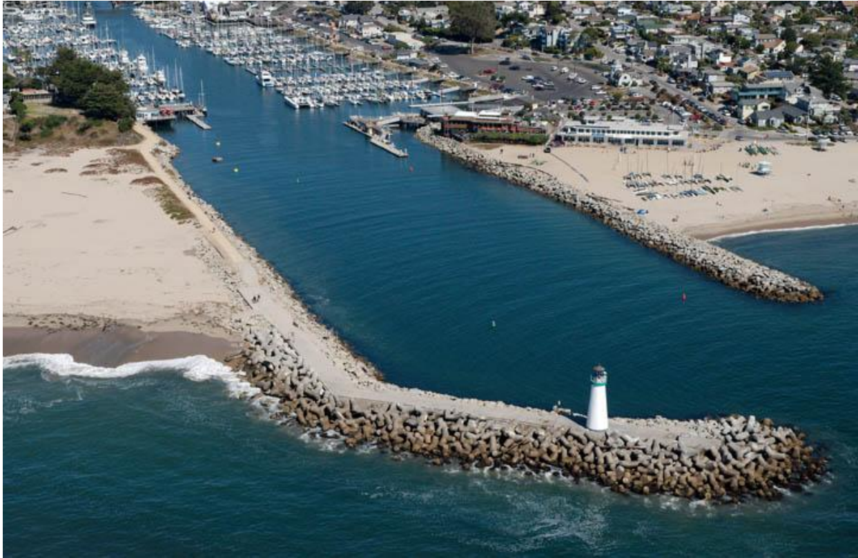
Figure 4-7. Aerial view of the two jetties that stabilize the entrance to Santa Cruz Harbor. Source Adelman and Adelman (2013)
