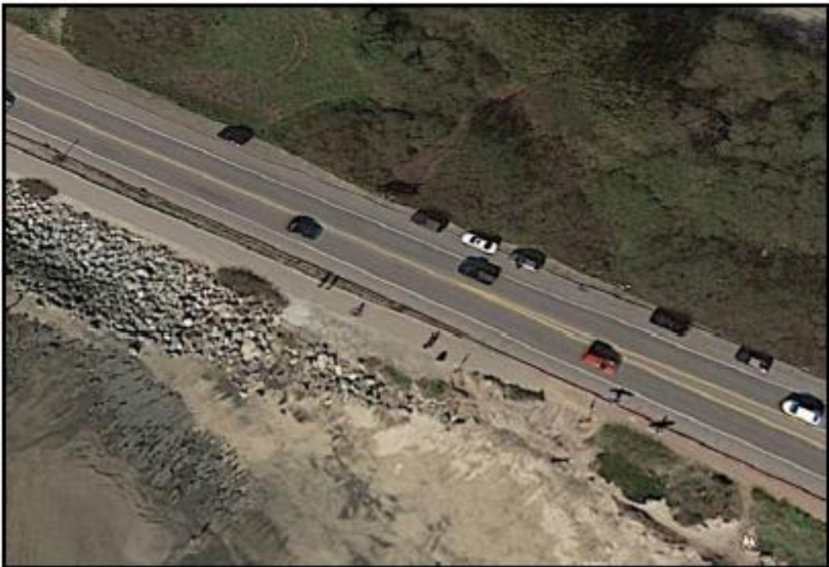
Figure 7-2. Vulnerable section of Highway 1 at Surfer’s Beach
