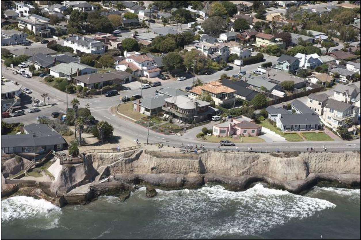
Figure 4-9. Aerial view of the recently completed East Cliff Drive Bluff Protection and Parkway Project. Source: Adelman and Adelman (2010)
