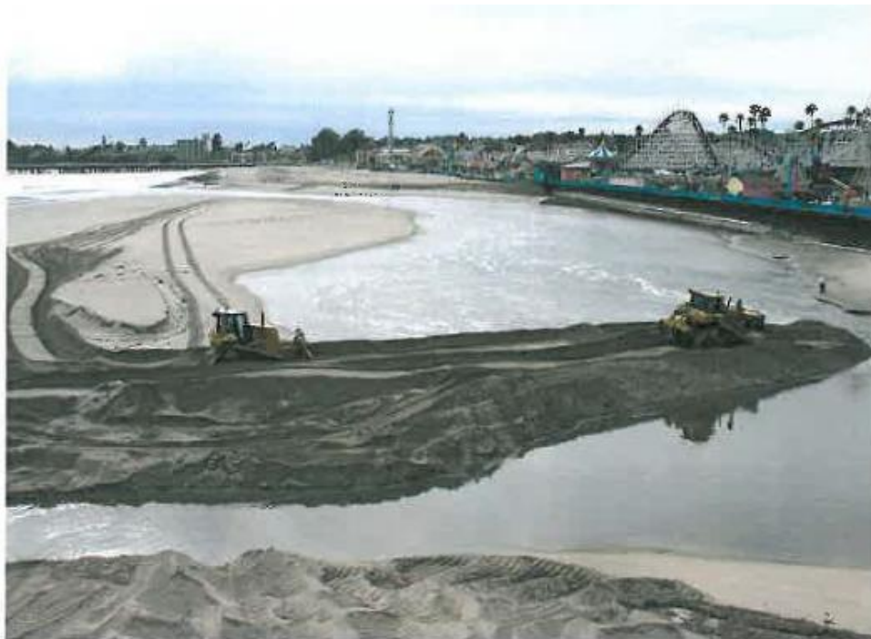
Figure 2-10. Emergency response to redirect the flow of the San Lorenzo River away from Santa Cruz Beach Boardwalk infrastructure (Source: Griggs, 2012)
