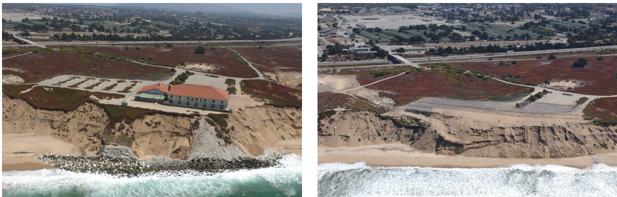
Figure 4-1. Stilwell Hall in 2003 and the site after demolition in 2004. Source: Adelman and Adelman (2003 and 2004)
