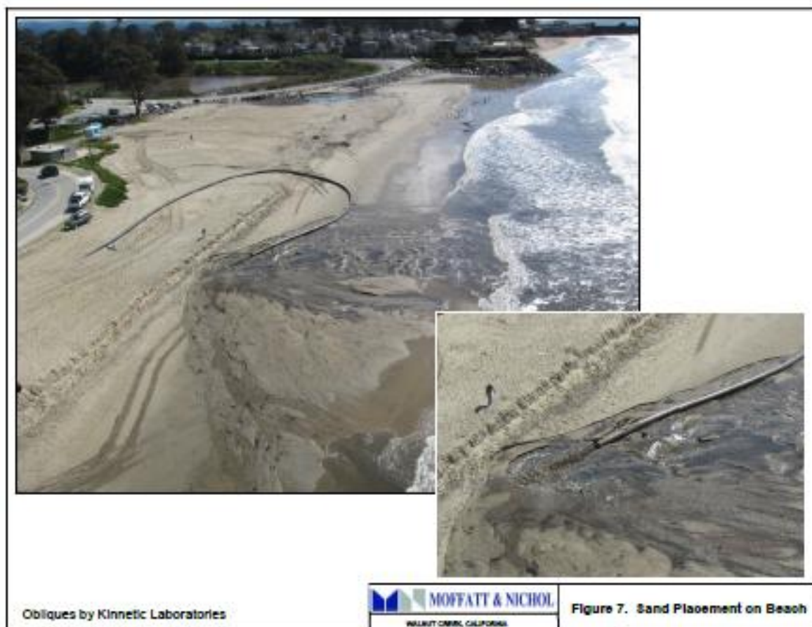
Figure 4-3. Beach nourishment operations at Twin Lakes State Beach. Source: Moffatt & Nichol et al., (2011)
