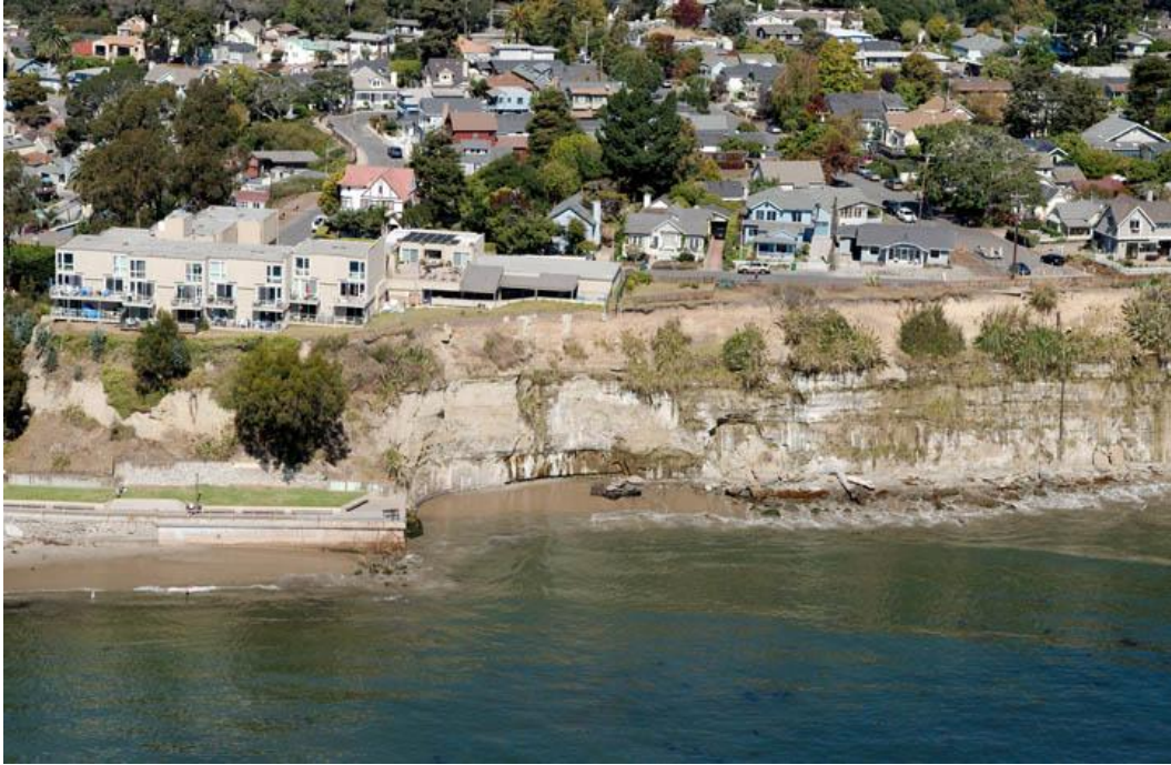
Figure 3-7. Aerial photograph of the western end of the Depot Hill BECA, dated October 2013. Note the significant sea cliff erosion, which threatens public and private infrastructure. Source: Adelman and Adelman
