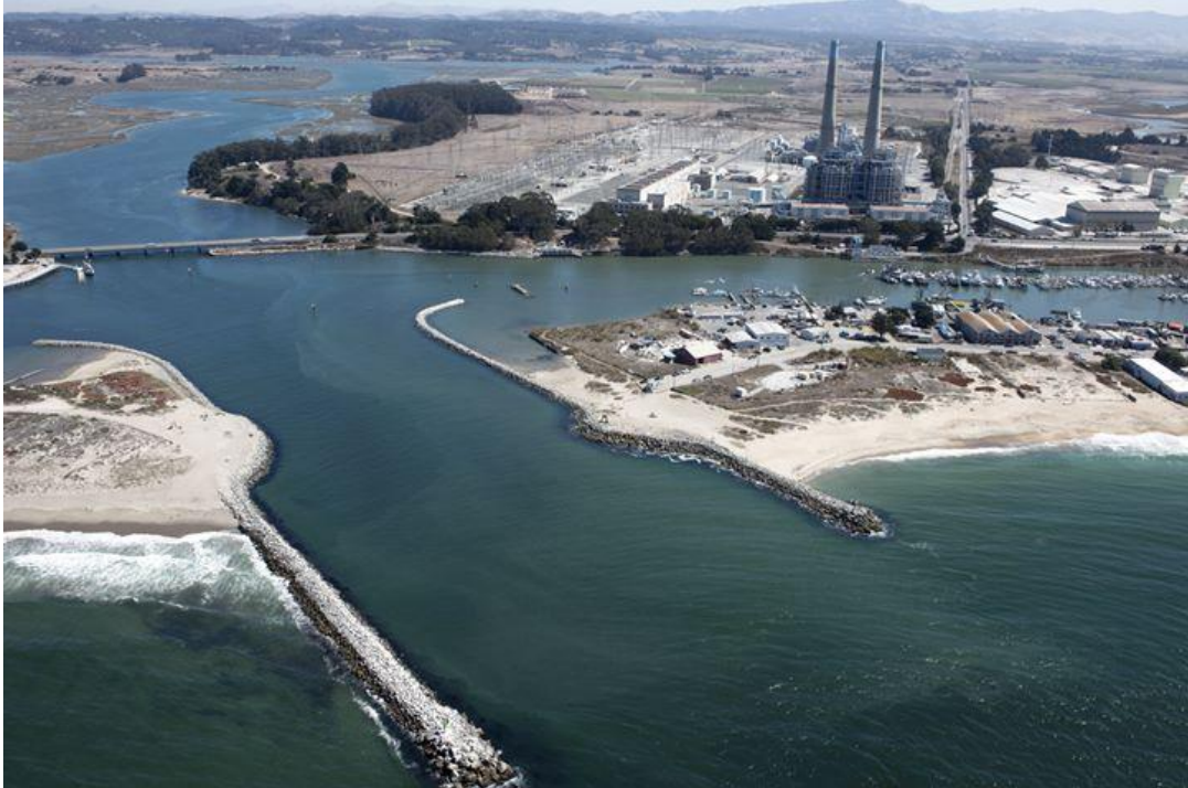
Figure 3-9. Aerial photograph of the entrance to Moss Landing Harbor and the Elkhorn Slough BECA (background), dated October 2013. Source: Adelman and Adelman
