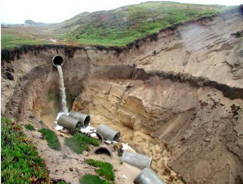
Figure B9: Storm drain outfall on Former Fort Ord compromised by coastal retreat. Waterfall undercuts weak sandstone substrate causing subsequent collapse of storm drain pipe sections. (see Fig. B9 for original location of outfall). Photo by David Norris September 2002. See Figure 18 for map view of the eroded canyon.
