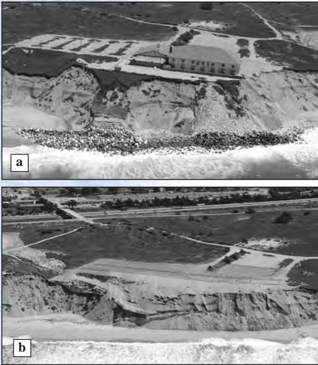
Figure 2. (a) August 2003 photograph of Stillwell Hall on Fort Ord in Marina (b) October 2004 photograph of the same site, after the building and riprap were removed because attempts to save the structure from collapsing into the ocean proved to be too costly and ineffective
